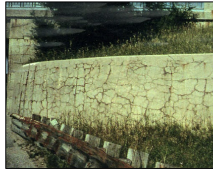
(b) Moderate ASR Cracking
