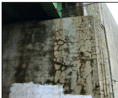
(c) Severe ASR Cracking
