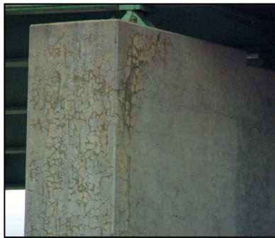
(a) Moderate ASR Cracking
